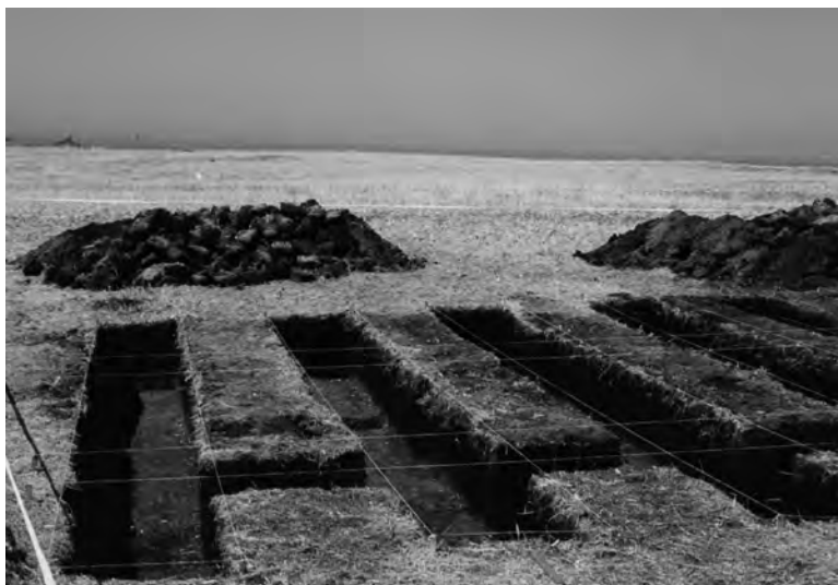
Figure 13.5 Systematically excavated trenches, and parallel cross-trenches, are an effective means to examine large areas of subsurface soil. The burial location of a U.S. Air Force RB-29 crewman, shot down over Yuri Island, Russia, in 1959, was readily identified using well-placed trenches that exposed the outline of the burial pit intruding into the undisturbed subsurface soil matrix.
