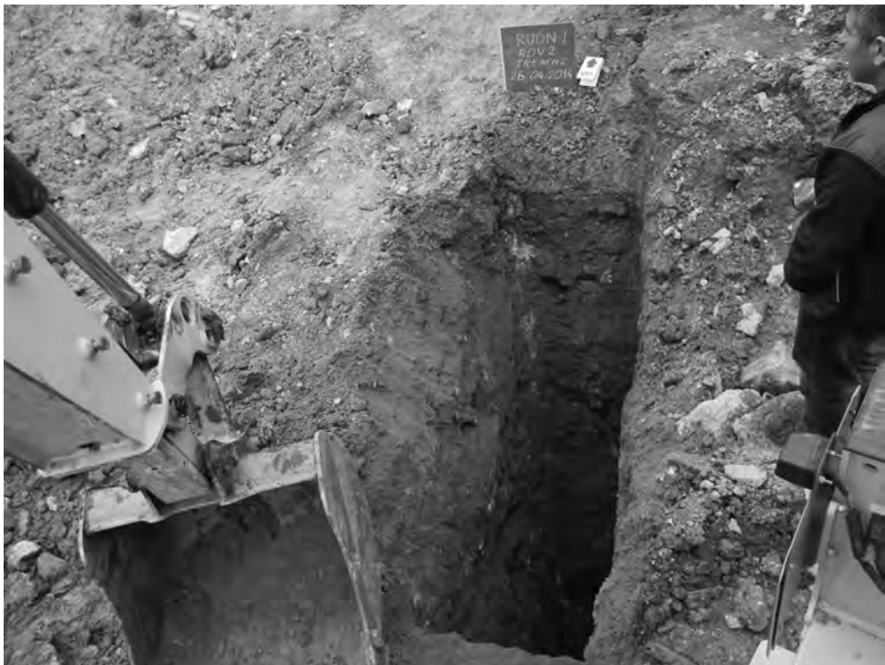
Figure 36.4 Series of deep control trenches excavated to check whether a house located on the site was intentionally built on the place where the bodies had been buried
