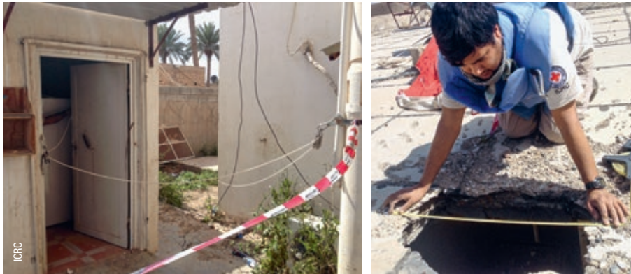
On the left, moving furniture semi-remotely, and on the right, a technical survey of a possible weapon entry point
