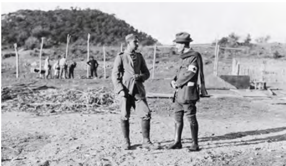
44. Oued Stita, Algeria. Camp for German prisoners of war. An ICRC delegate speaks to the prisoners' spokesman. The camp is still under construction, and the first step is to erect the fence.
