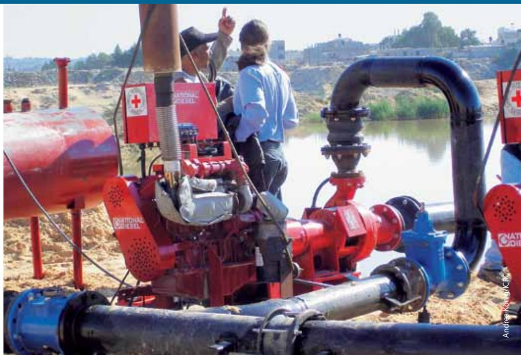
Emergency pumping system being set up in Beit Lahia to prevent the banks of a wastewater reservoir from bursting
